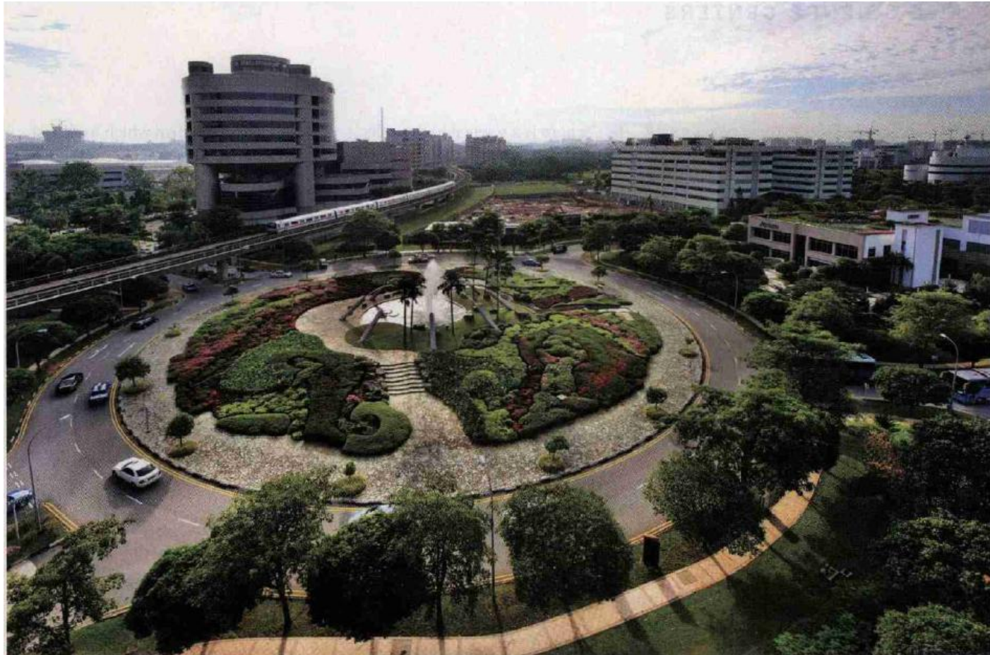
Photo courtesy of JTC Corp.
